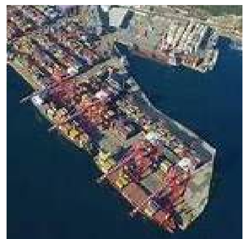
YILPORT PANAMA PORT PROJECT
