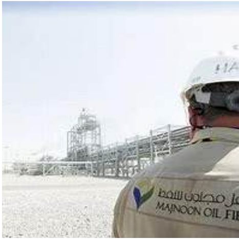
MAJNOON132/33KV GRID SUBSTATION BASRA OIL COMPANY (BOC)
